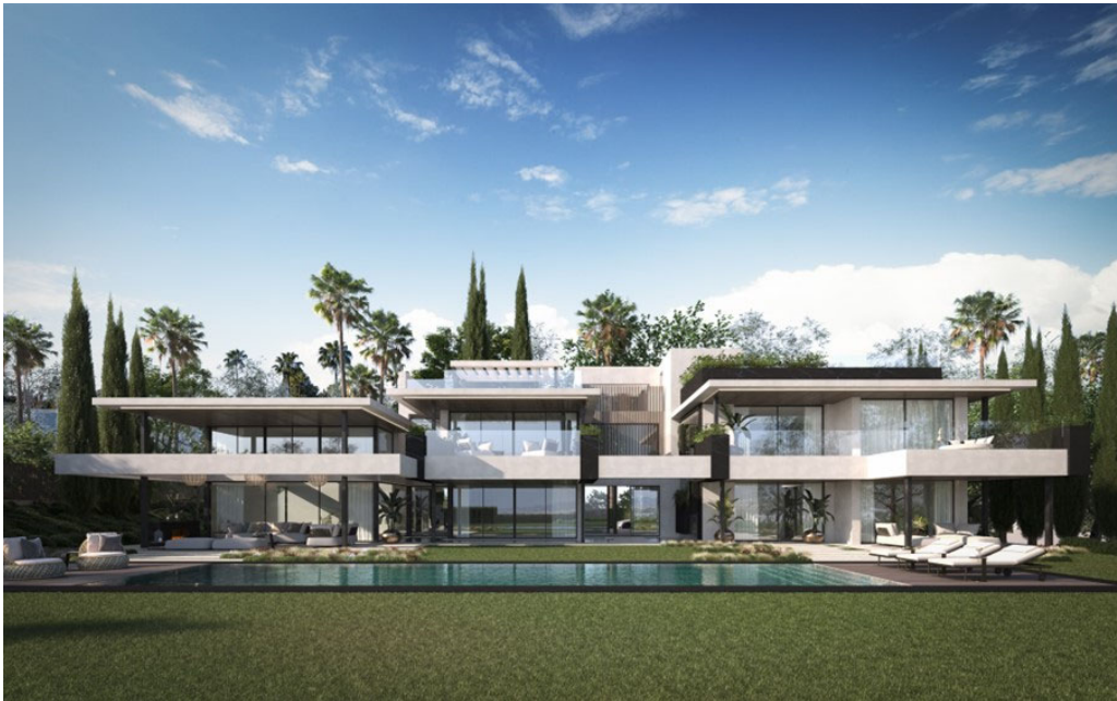
Façade facing the garden of the villa.
