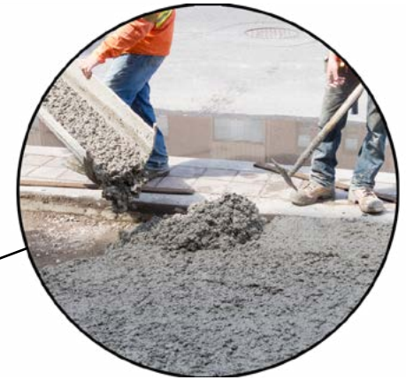
Concrete Foundation of concrete: HA-25/B/40/IIa
