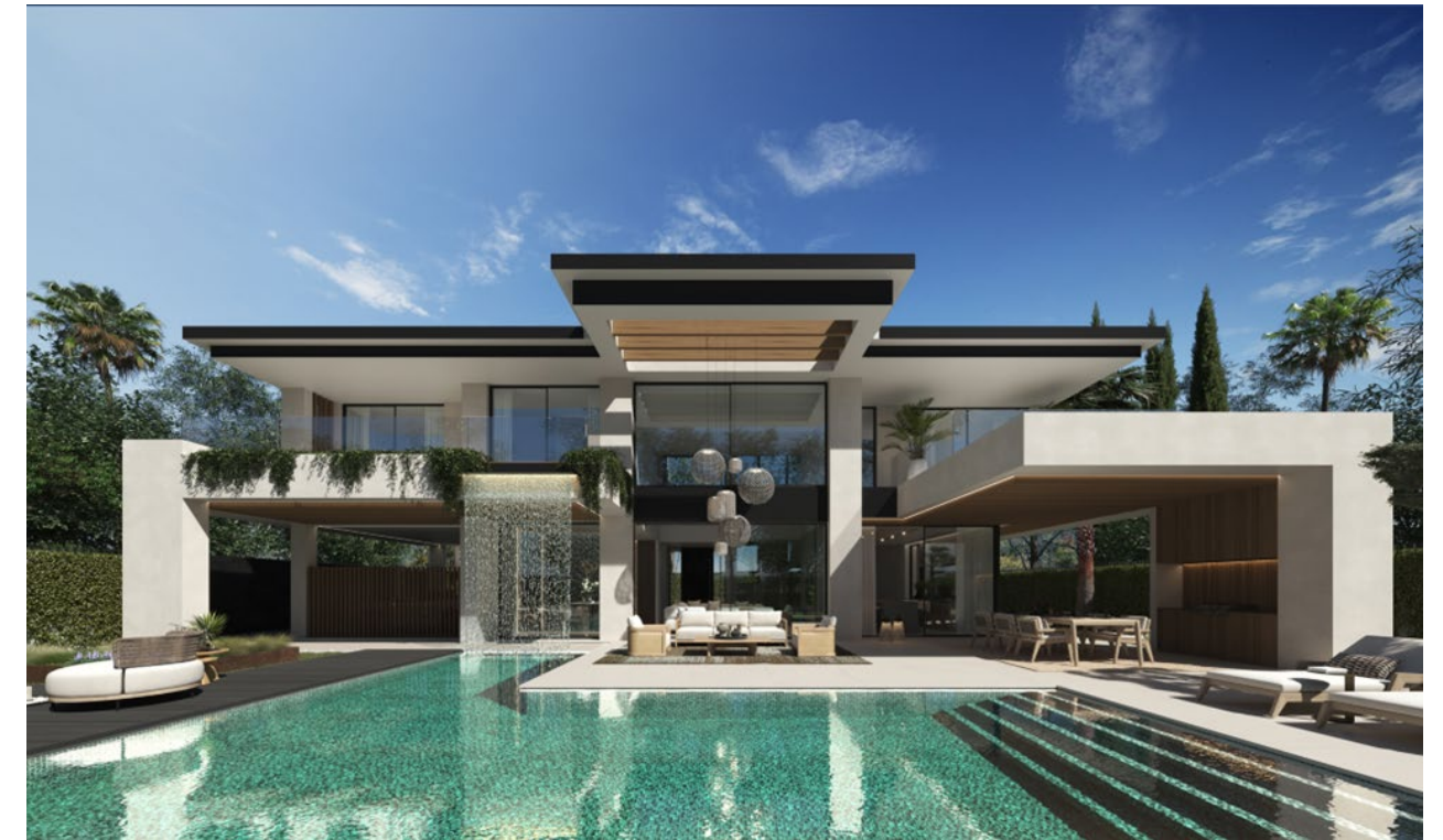
Façade facing the garden of the villa.
